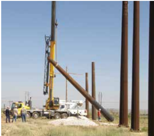
Transmission poles being set.
